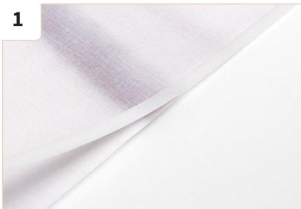
Stick an adhesive connector tape to the back of each panel at both the upper and lower end.
